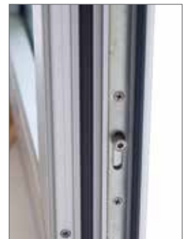
Locking Roller Mechanism for Multi Point Locking Systems – Standard
